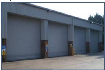
Activation Options: As our standard offering opening activation on electric shutters is "dead man down" operation, i.e. the operative needs to keep their finger on the button to lower the door. Various automated activation options are available, such as radar, remote control and floor laid vehicle detection loops. Each require the addition of safety beams and a safety bottom bar that can be supplied factory fitted.
